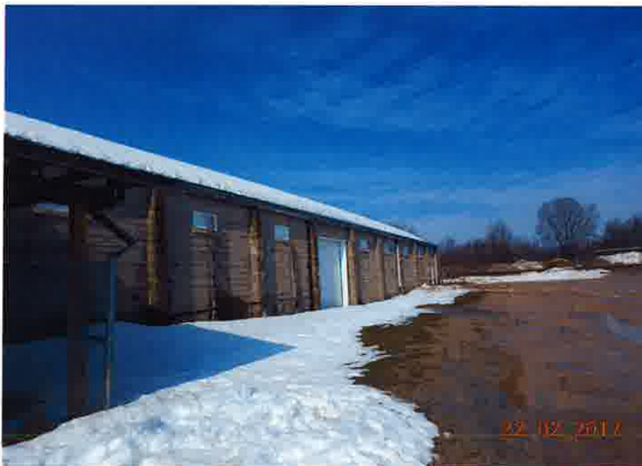
Photo 4: View from the southwest.
